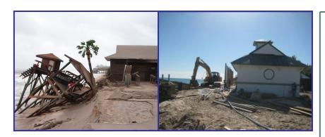
In September 2004, Hurricanes Frances and Jeanne severely damaged Wabasso Beach Park. The storms destroyed the boardwalk, restroom, pavilions and portions of the parking area and roadway within the Park. Work by Coastal Tech entailed coastal engineering design, permitting and construction phase services to provide for restoration of the Park.
